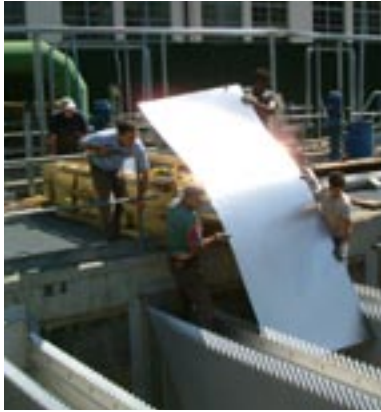
Installation of lamella plates at Como WWTP, Italy.
