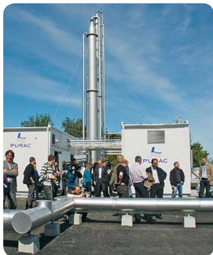
Stavanger, Norway, 500 Nm 3 /h, 300 scfm.
